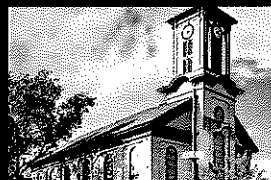
Clock Tower at Simpson United Methodist Church (circa 1866) 331 High St.
